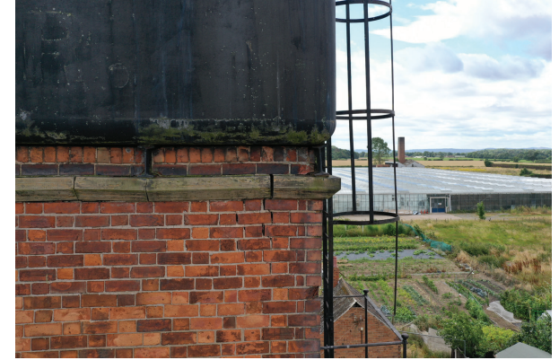
North elevation, movement & damage to the brickwork and corbel at the west end
