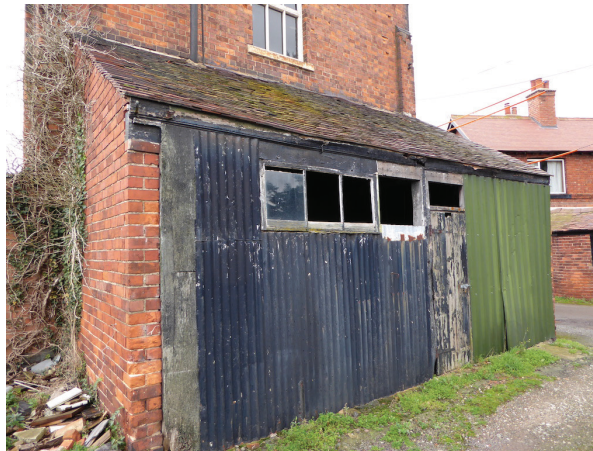
South lean-to: brick gable walls, corrugated metal walls and tiled roof
