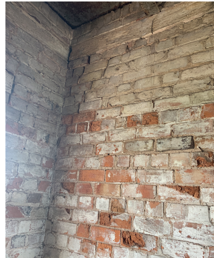
Internal condition of the brickwork, note cracking to corners
