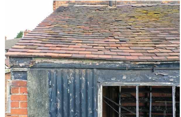
Dilapidated condition of the south lean-to, both the walls and roof tiles
