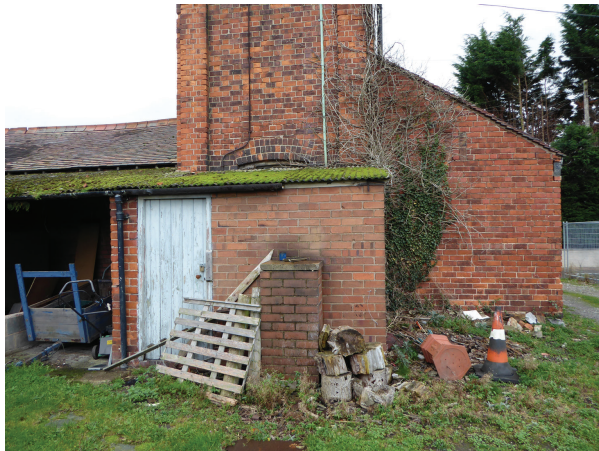
The 'pump house' later addition lean to at the west end - note the partially covered window on the original west elevation
