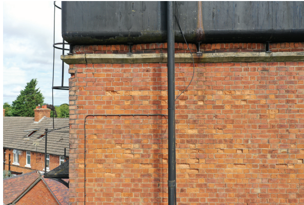
Deteriorated brickwork to the south elevation
