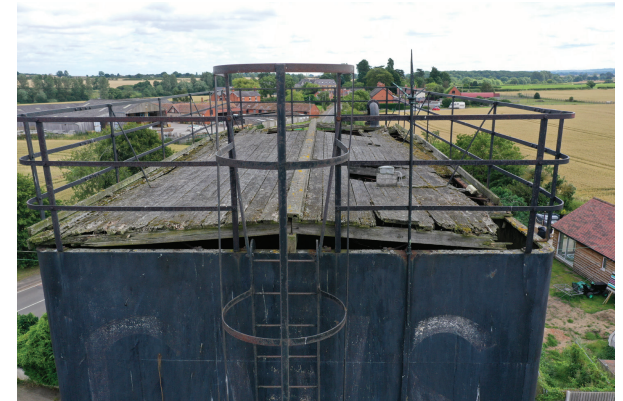
Existing timber 'roof' to the water tank, view from the west
