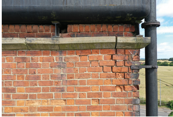
South elevation, movement and associated damage at the east end
