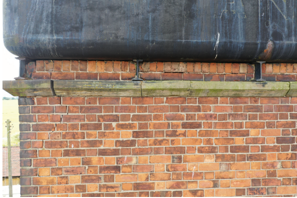
South elevation, damage to the brickwork and stone corbel at the west end
