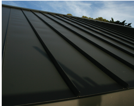
Example of metal standing seam roof
