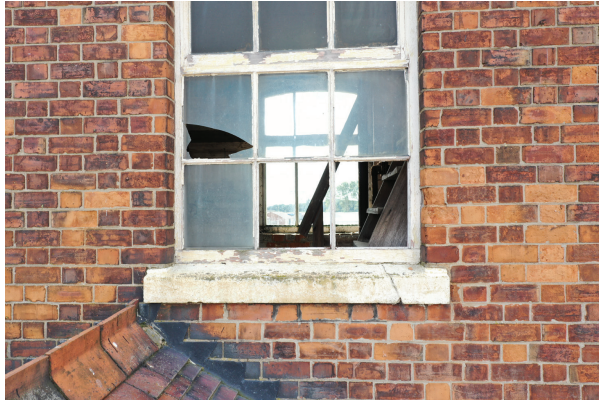
Damage to the timber window within the north elevation
