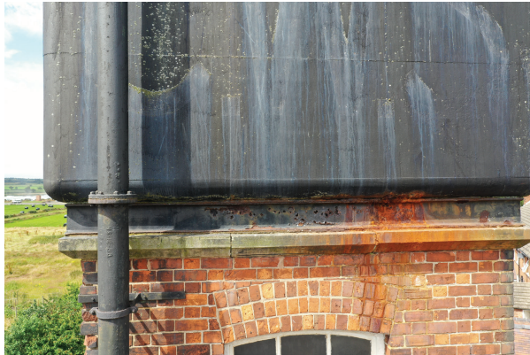
East elevation, damage to the steel and corbel under the water tank
